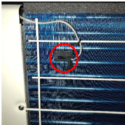
(Amb. Air temp sensor, Plastic seal)
